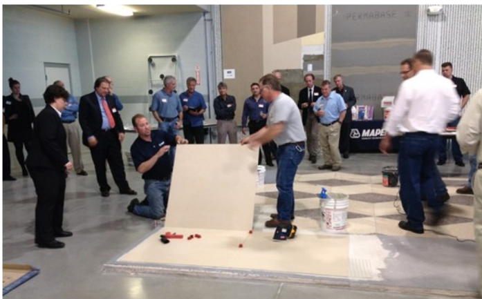
BAC Tile Representative Bill Breheny demonstrates laying large format thin porcelain tile at a meeting of the Ceramic Tile Contractors Association of Chicago held at the IMI training center in Addison, Illinois.
